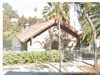
LA SAN currently maintains (1/22) restrooms near high traffic zones
