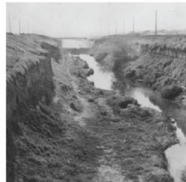
Alondra Boulevard Compton Creek Bridge, 1947
