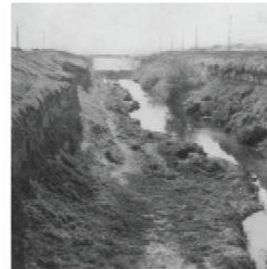
Alondra Boulevard Compton Creek Bridge, 1947
