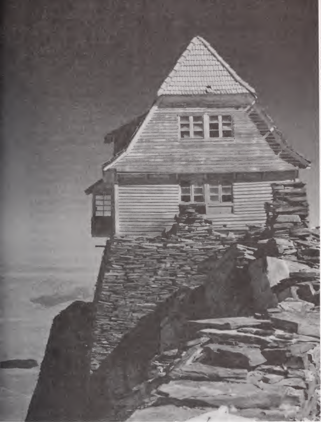
A ski lodge building on Chacaltaya (elevation about 5,500 meters) near La Paz Courtesy Harvey W. Reed
