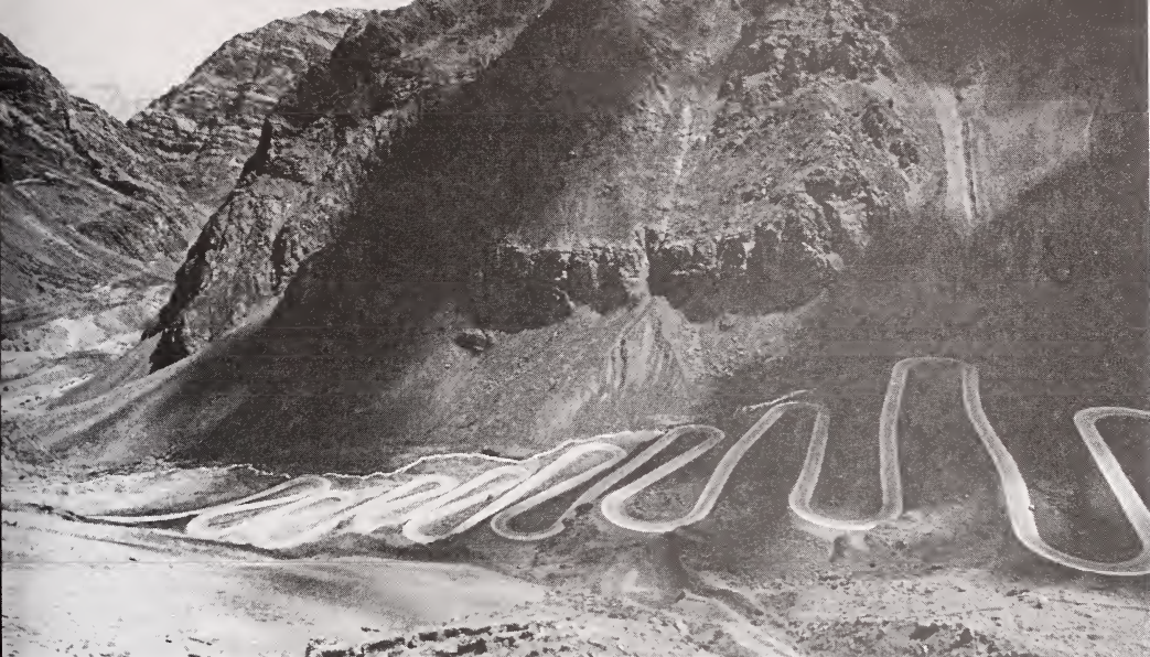
A view of the Trans-Andean Highway, the most important road link between Argentina and Chile Courtesy Inter-American Development Bank
