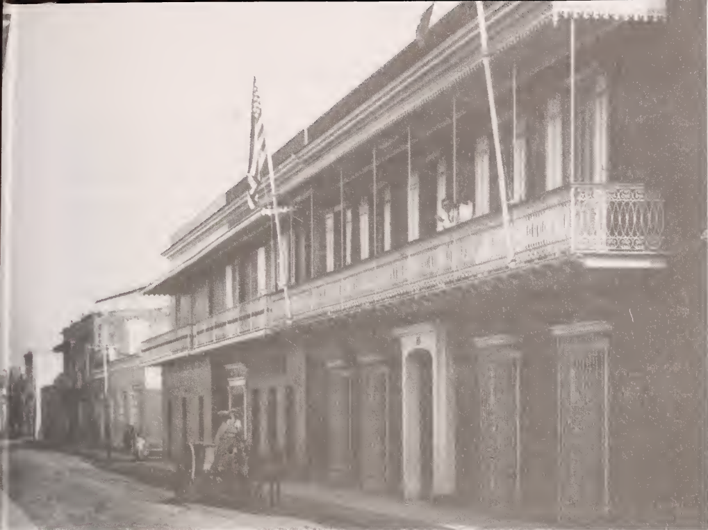
Offices of the General Customs Receivership, Santo Domingo, 1907 Courtesy National Archives
