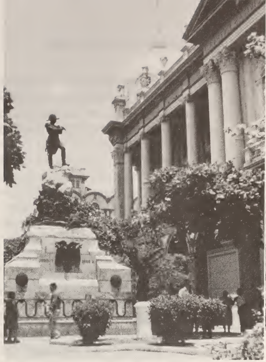
Municipal building, Guayaquil Courtesy Embassy of Ecuador, Washington
