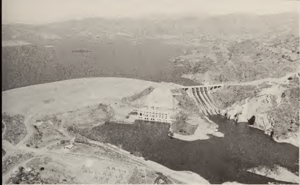
Cerrón Grande hydroelectric project, northwestern El Salvador Courtesy Inter-American Development Bank
