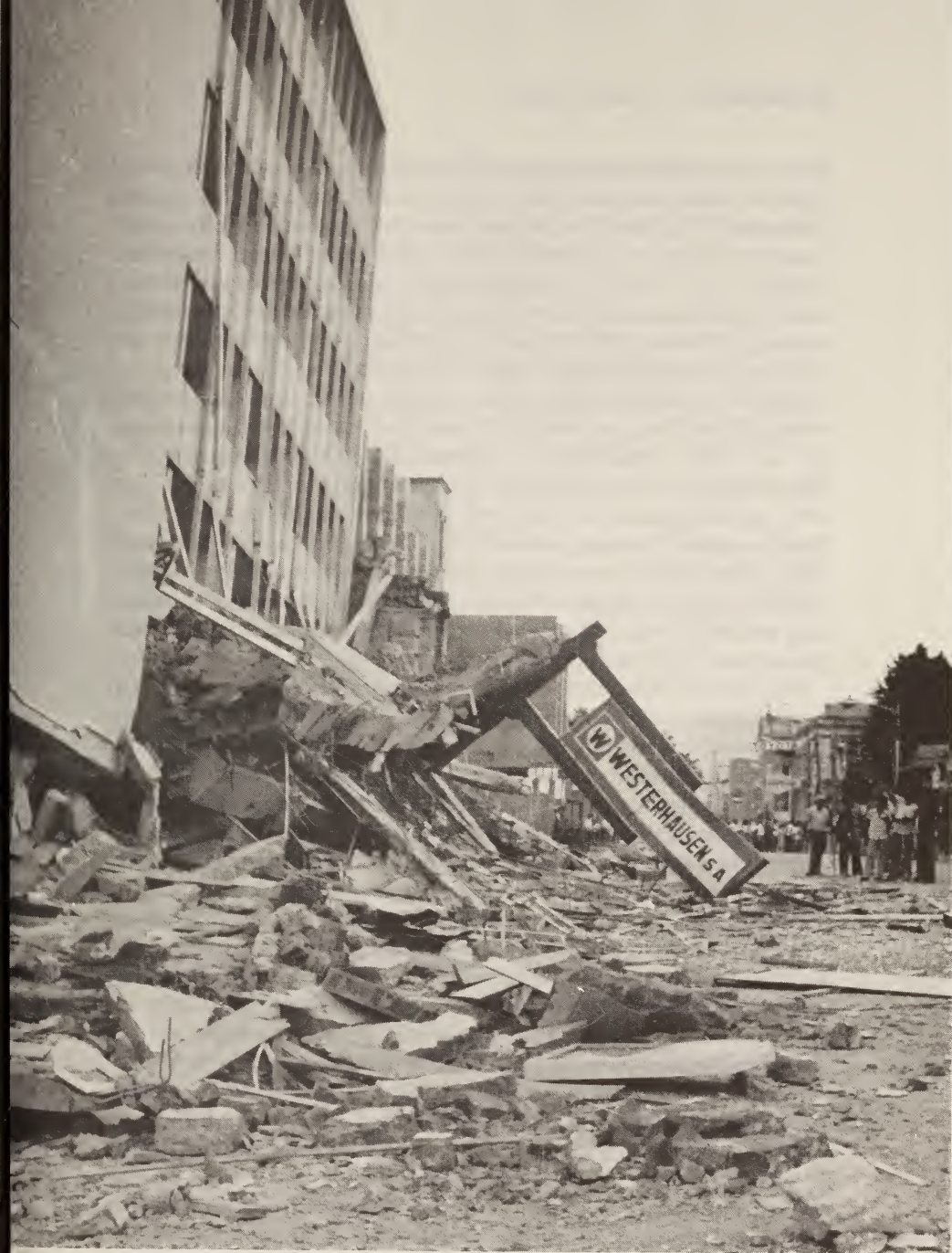
Earthquake damage, San Salvador, October 1986 Courtesy Inter-American Development Bank
