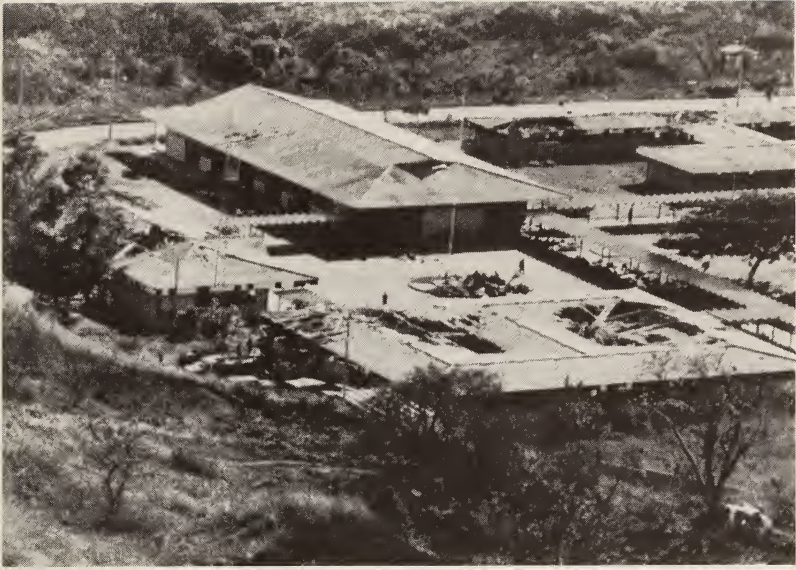
Damage to Fourth Infantry Brigade compound from guerrilla attack, El Paraíso, Chalatenango Department, December 1983 Courtesy United States Department of Defense
