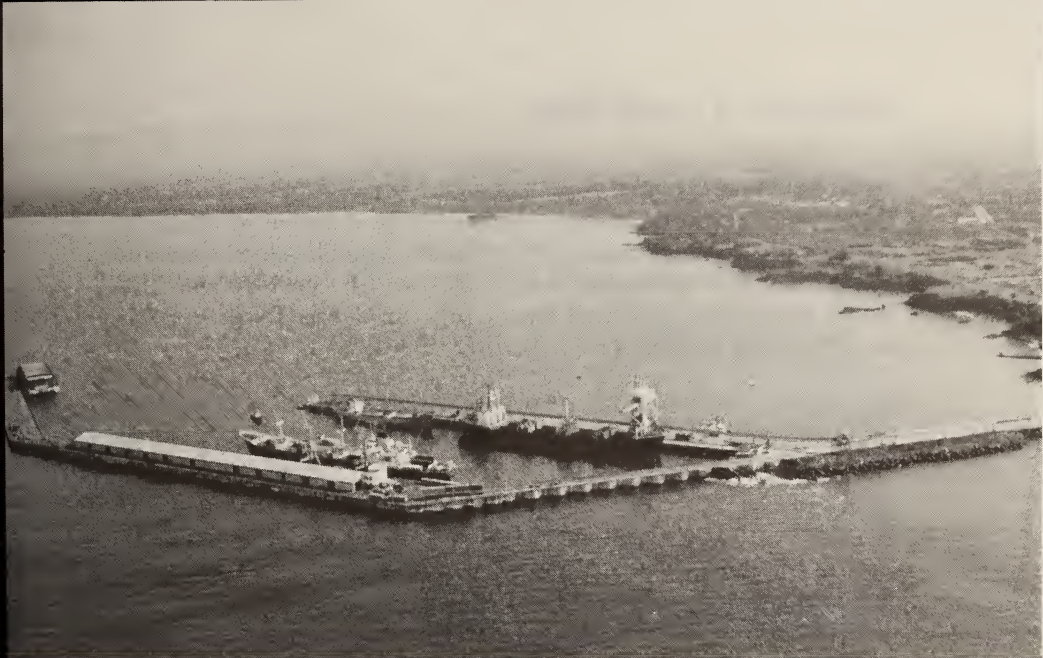
Port expansion at Acajutla Courtesy Inter-American Development Bank
