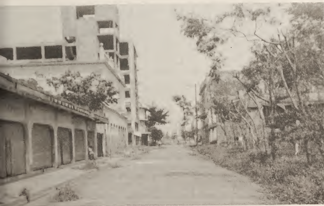
Many buildings in downtown Managua, damaged in the 1972 earthquake, remained unrepaired in 1993. Courtesy Edmundo Flores
