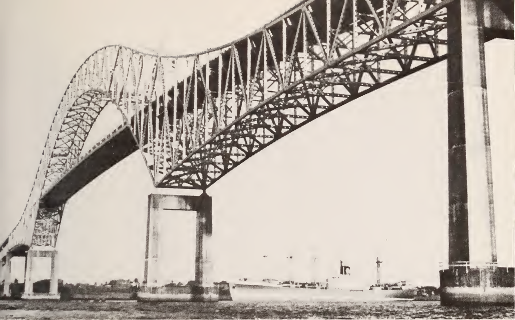
Thatcher Bridge over Panama Canal Courtesy Pan American Union
