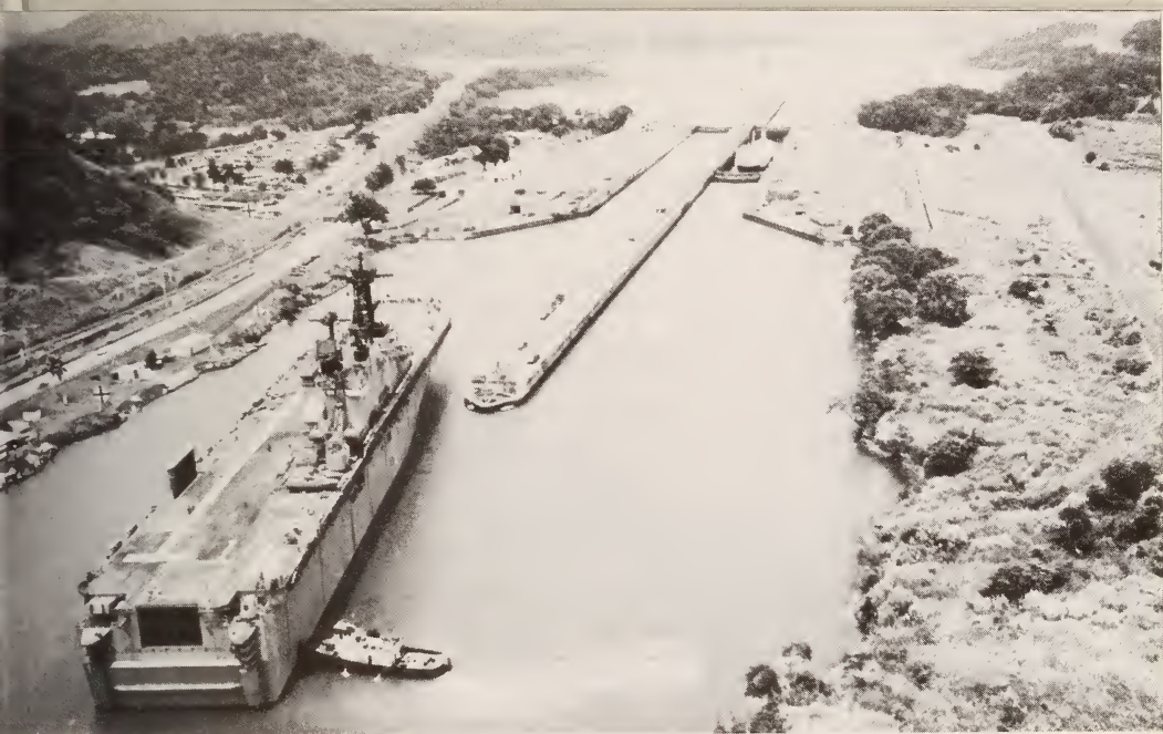
U.S.S. Tarawa enters Pedro Miguel Locks, Panama Canal, July 1976 Courtesy Agency for International Development
