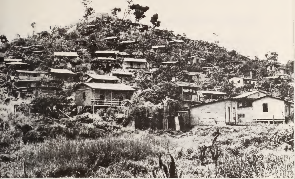
Squatter dwellings in San Miguelito Courtesy Agency for International Development
