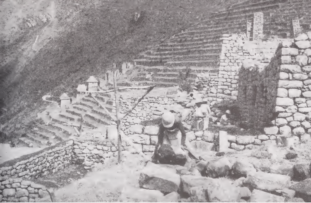
Workers repairing a military section in Machupicchu Courtesy Inter-American Development Bank
