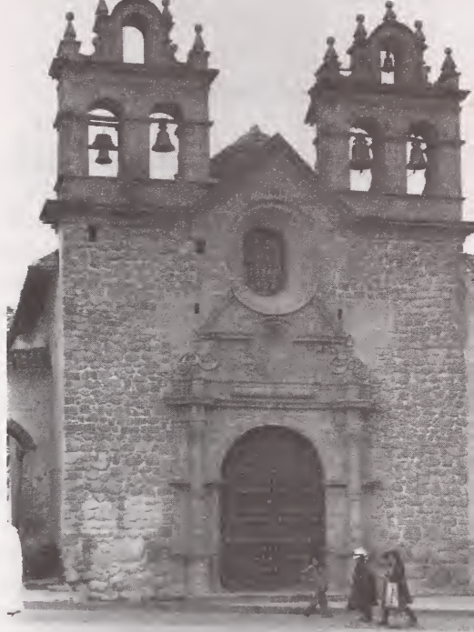
Church of San Antonio Abad in Cusco Courtesy Inter-American Development Bank
