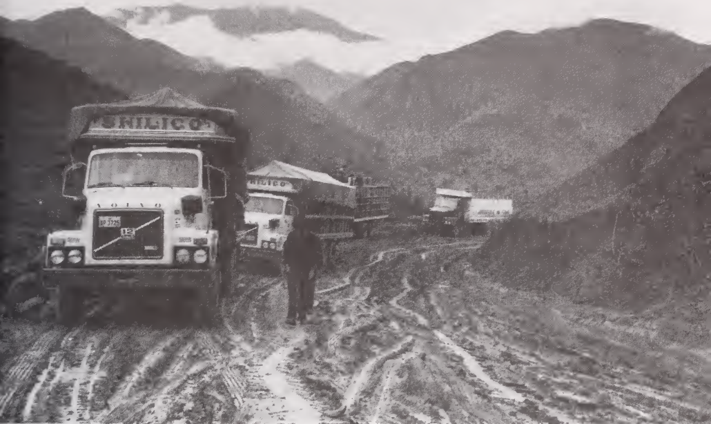
Trucks passing a construction area on the northern coast-to-jungle Olmos-Corral Quemado road Courtesy Inter-American Development Bank
