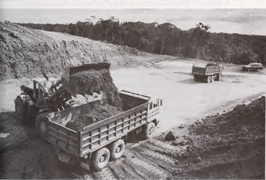
Siderúrgica del Orinoco (Sidor) steel mill Courtesy Inter-American Development Bank Loading bauxite ore, Los Pijiguaos Mine, Bolívar State Courtesy Inter-American Development Bank
