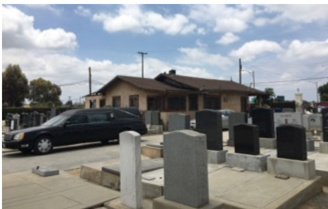
Figure 4.19: Current Beth Israel Service Building. Photo by author.
