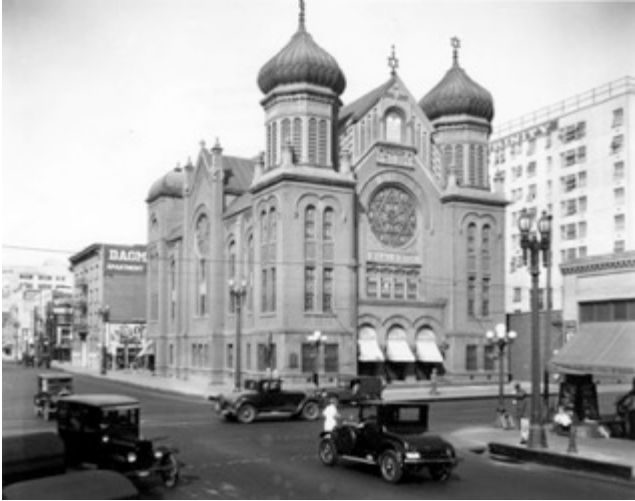
Figure 1.1: B'nai B'rith Congregation's second synagogue at the corner of Ninth and Hope streets, 1926. Courtesy of the Security Pacific National Bank Collection/Los Angeles Public Library; image 00081601.
