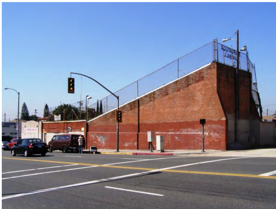
Figure 1.1: Maravilla Handball Court. Photo by ASM Affiliates. Source: “Maravilla Handball Court and El Centro Grocery Store,” Los Angeles Conservancy, accessed January 5, 2018, https://www.laconservancy.org/issues/maravilla-handball-court-and-el-centro-grocery-store .
