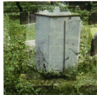
Fig. 5. Emergency stabilization using a closed, ventilated box around the structure. Photograph by Frank Matero.
