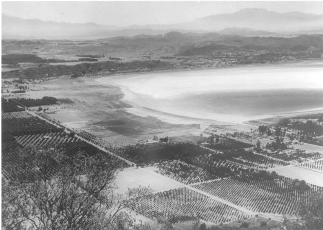
Figure 38. West end of Lake Elsinore and Riverside Drive from the Ortega Highway circa 1950s. Today most of the area shown in this photograph has been converted from agricultural land to planned community subdivisions. The town center is in the background on the edge of the Lake towards the right. Lake Elsinore Public Library Collection.
