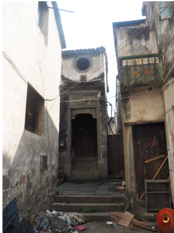
Figure 4.4: Potential Historic Grand Taimen Comfort Station Site
