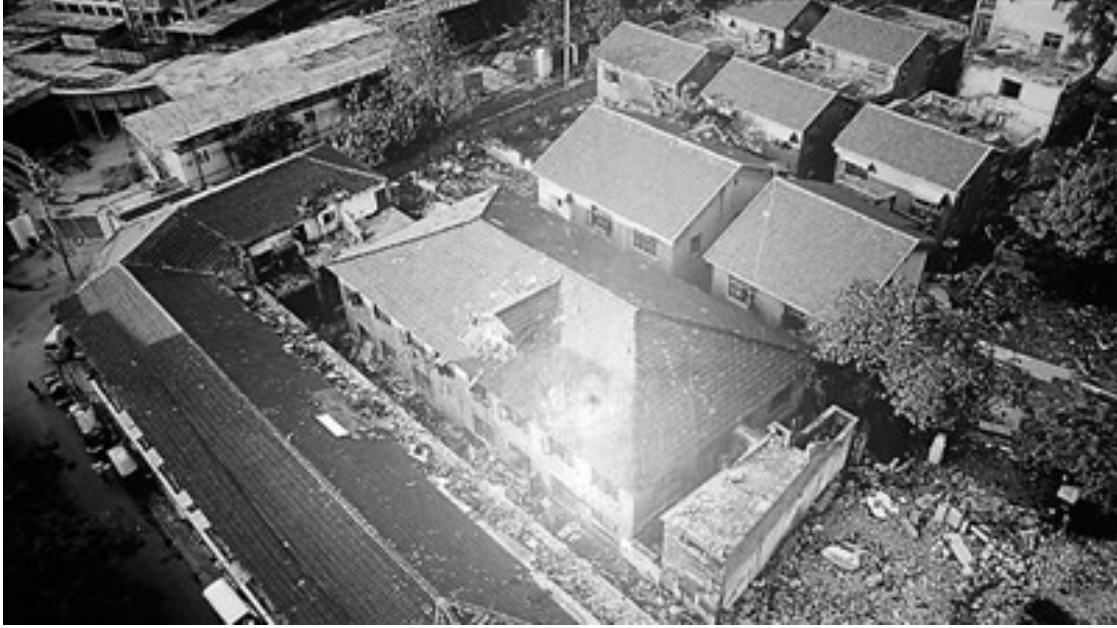
Figure 3.7: Historical Photo of Nanjing Liji Lane Comfort Station
