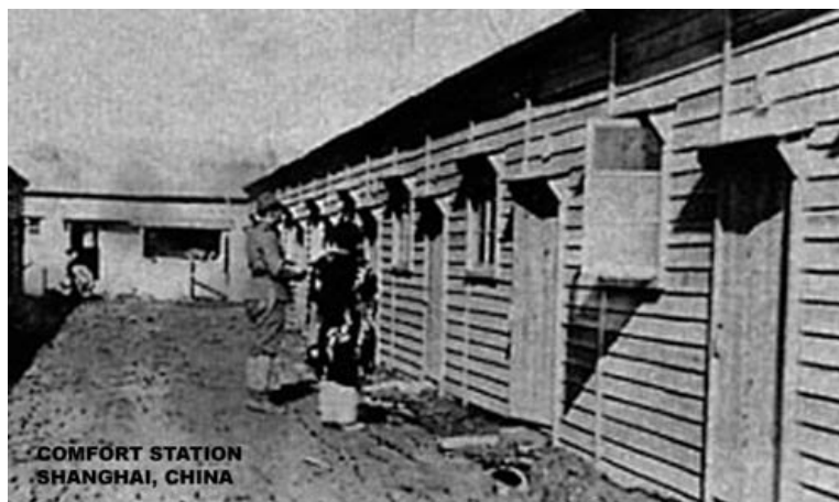
Figure 2.6: Comfort Station in Yangjiazhai, Shanghai
