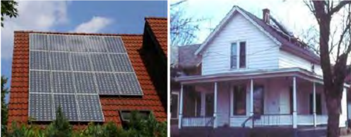
Fig 1.2: Solar roofs installations examples; left figure shows solar panels on a rear roof, the right figure shows a wrong installation - the solar panels are visible from the public right-of-way. Source: Oklahoma City Historic Preservation Design & Sustainability Standards and Guideline.
