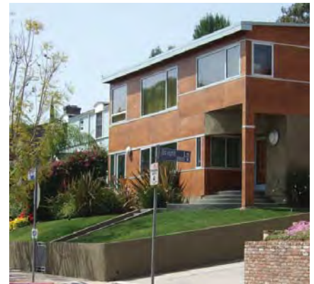
Though innovative and interesting, the materials on this home do not relate to those used in its surroundings.
