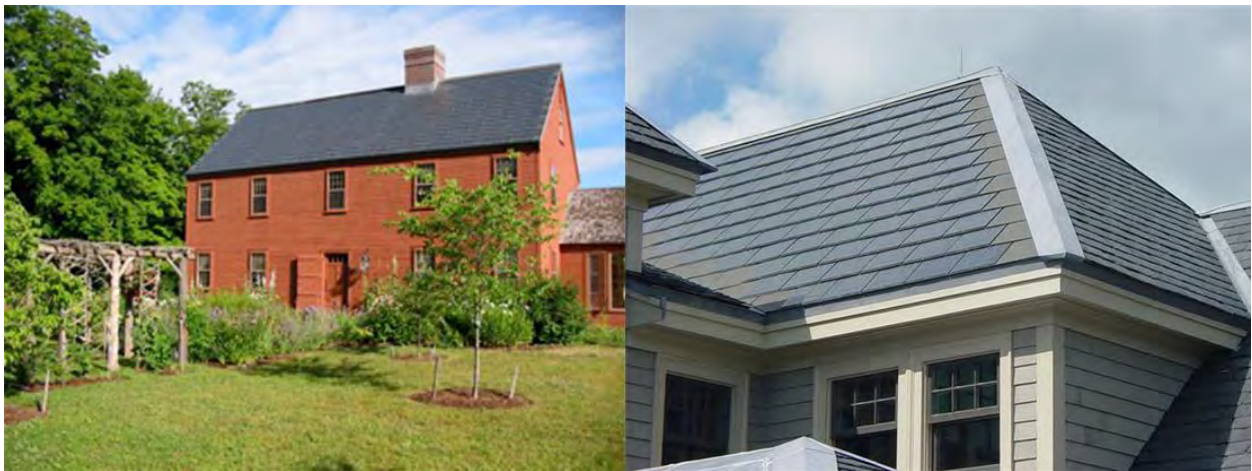
Fig 2.3: Solar roofs installations on some residential houses; left figure is a red house in Bolton, Massachusetts, right figure is a house with solar slates in Falmouth, Massachusetts. Source: provided by Aesthetic Green Power from email.
