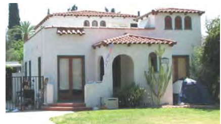
This second-story addition is set-back and preserves the look and scale of the original bungalow.
