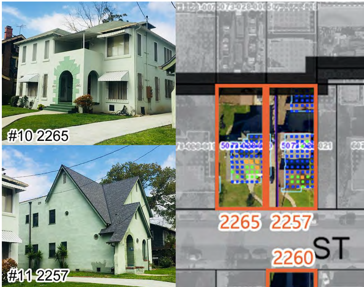
Fig 5.8: Photos show #10 and #11 properties with their solar maps. The solar maps indicate solar access on front roofs. Yet, according to preservation plan that “solar panels should not be placed upon rooftops that are visible to the general public”, it will be inappropriate to install solar panels on the front roofs of these two properties. Sources: Photos by author, the solar maps are based on L.A. County Solar Map.
