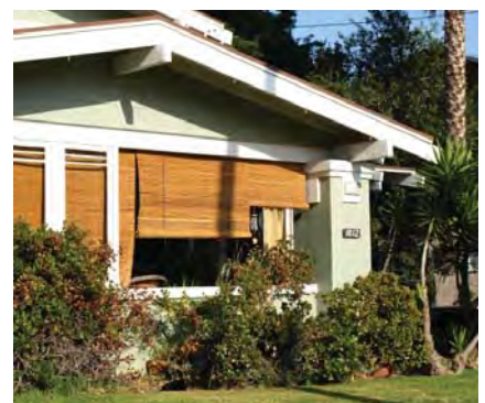
Non-permanent devices such as this bamboo screen may effectively screen a porch without altering the home and disrupting the streetscape.
