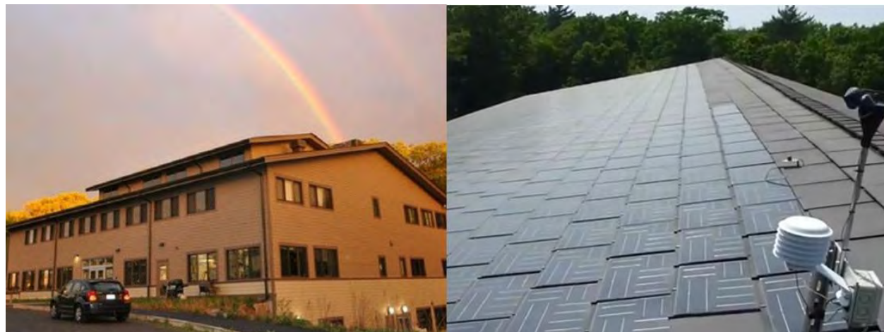
Fig 2.4: The New England Wildlife Center's green building in Massachusetts. Solar roofs have produced five percent of total building energy. Source: "Our Green Building," New England Wildlife Center, https://www.newildlife.org/about-2/green-building/ , photo rights authorized by e-mail.
