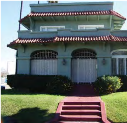
Enclosing a front porch disrupts the porch's intended purpose as an outdoor room.
