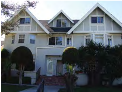
The modern windows that have been added to this home are poorly scaled and dramatically alter the home's original appearance.
