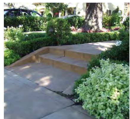
Poured concrete steps and walkways are a common feature in the neighborhood.
