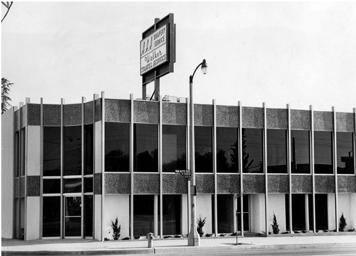
Figure 2.12: 1965 New Plant for Virgil Walker's AAA Drapery Service and Walker Travel Agency, 13460 Van Nuys Blvd. The building would later become the home of the MEND, a community organization providing aid and services to underprivileged community members. Source: Valley Times Collection, Los Angeles Public Library.
